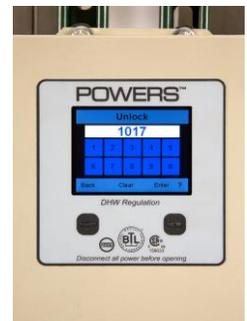
Most systems are also field-configurable without the need for a laptop or special software. Digital water mixing and recirculation can easily be integrated into a building automation system (BAS) to allow facility managers to remotely monitor and control water temperatures.
